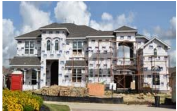
Single-Family Home Under Construction (MUD 502)
