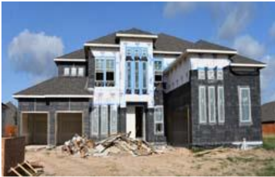
Single-Family Home Under Construction (MUD 501)
