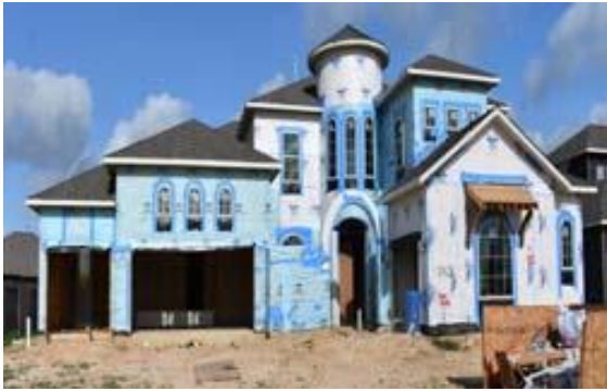
Single-Family Home Under Construction (MUD 501)
