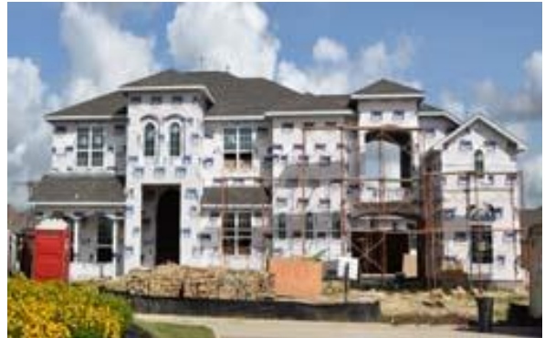
Single-Family Home Under Construction (MUD 502)
