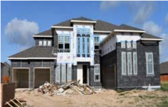
Single-Family Home Under Construction (MUD 501)
