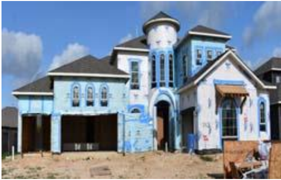
Single-Family Home Under Construction (MUD 501)
