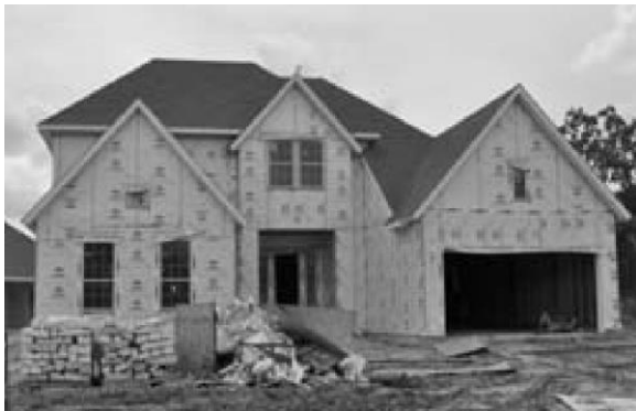
Single-Family Home Under Construction
