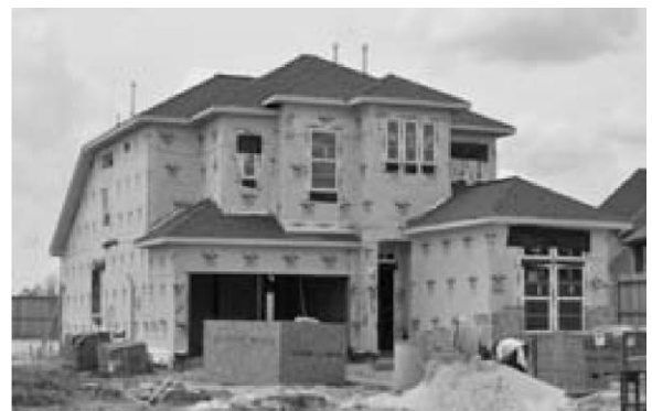
Single-Family Home Under Construction
