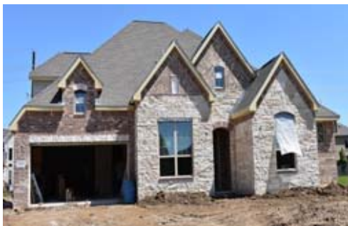
Single-Family Residential Under Construction
