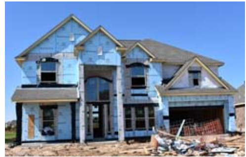
Single-Family Residential Under Construction
