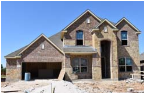
Single-Family Residential Under Construction
