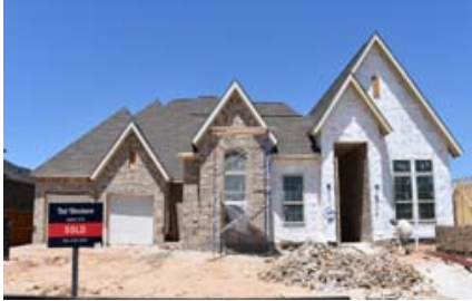
Single-Family Residential Under Construction
