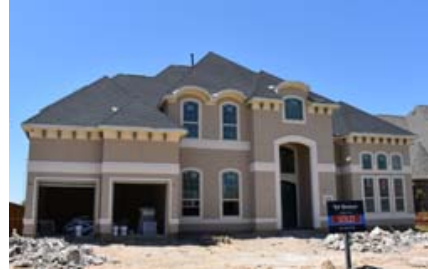
Single-Family Residential Under Construction
